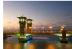
Stanley bridge, Alexandria, Egypt
