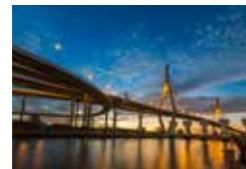
The Rama VIII Bridge, Bangkok, Thailand
