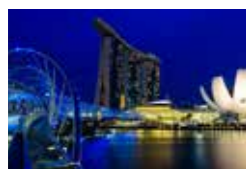
Helix bridge Singapore, Republic of Singapore
