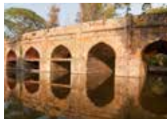
Athpula Bridge, Lodhi Gardens in Delhi, India
