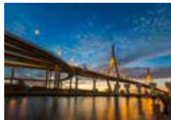
The Rama VIII Bridge, Bangkok, Thailand
