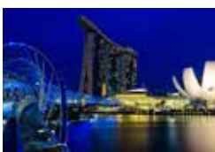
Helix Bridge Singapore, Republic of Singapore
